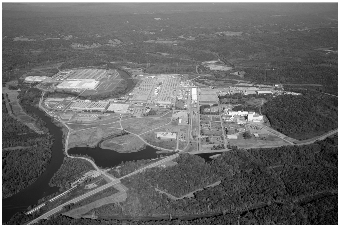
Fig. 1.10. East Tennessee Technology Park.
